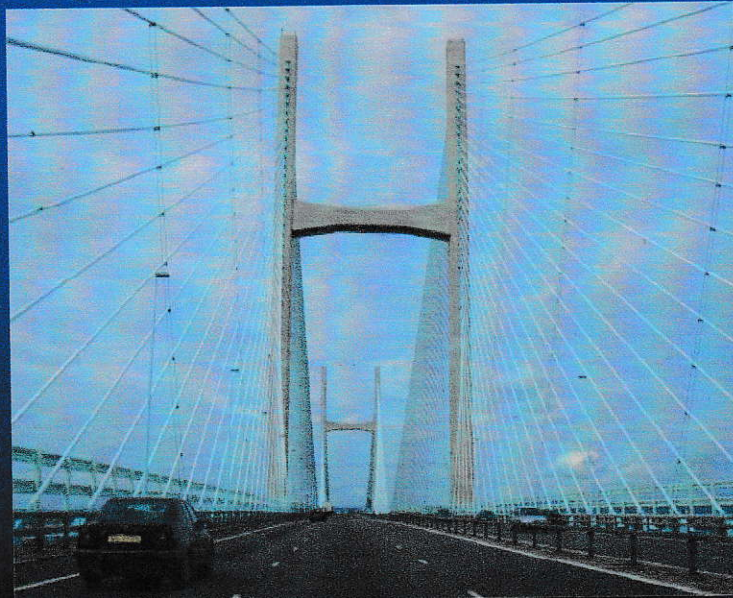
Bridge over River Severn: Second Crossing: 1996
