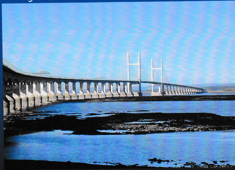
Bridge over River Severn: Second Crossing: 1996
