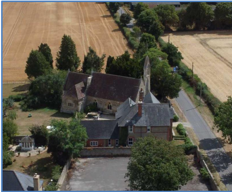
The building of St James' church at Bourton (Berks Chronicle 13 th August 1859)
