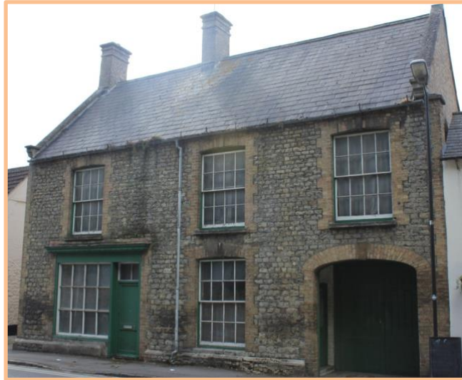
The premises that was the Bakery used by Crusty Fuller, 1900 - 1922, now skilfully renovated by the current owners
