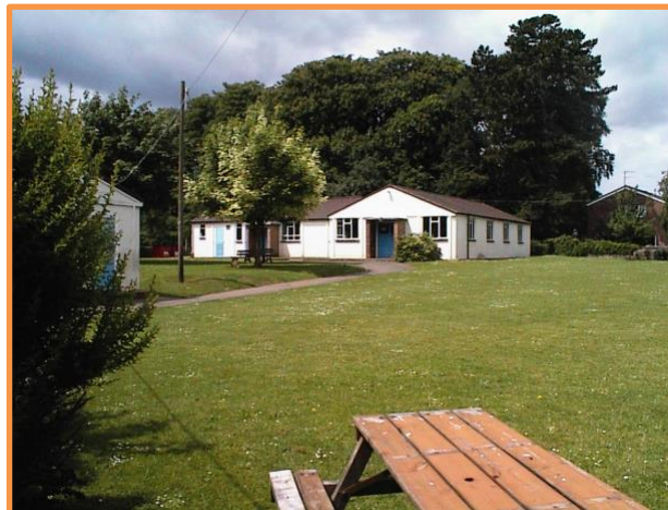
The old The pre-fab building that was the Kitchen, Dining Room and Assembly Room. Now gone. Photo by Neil B. Maw
