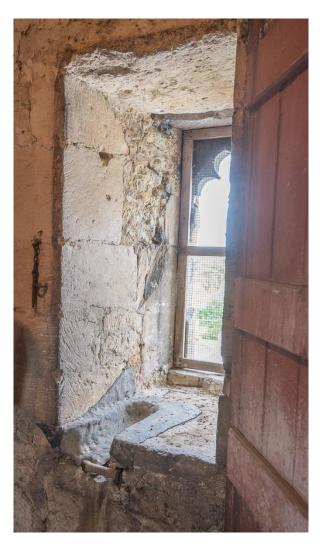
Here a deep groove is worn in the sill of the East of the windo. The sanctus bell once stood in this window and its rope pulled over the sill.
