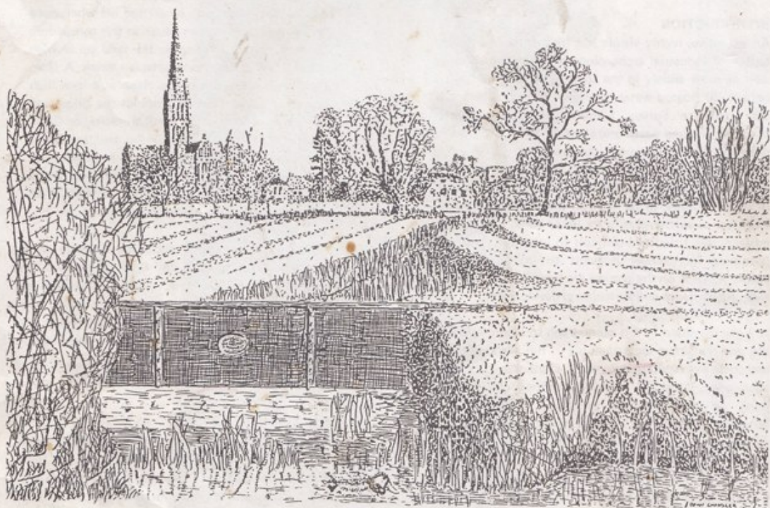
Cast iron sectional aqueduct, part of the West Harnham system.
